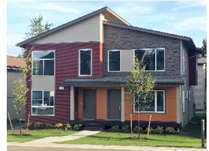
Good site access for pedestrians.
