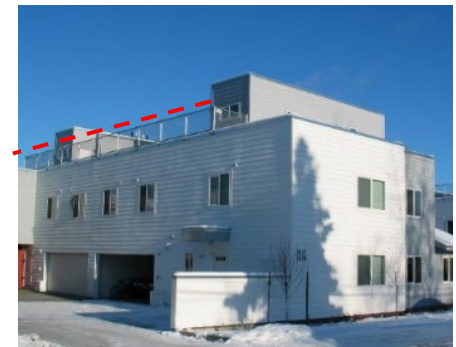
Rooftop Parapets, Stairwells
